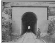
Tunnelville tunnel, La Farge, 1900. La Farge Public Library/Winding Rivers Library System
